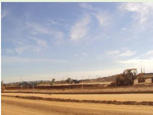
Figure 2: Construction activity seen on site
